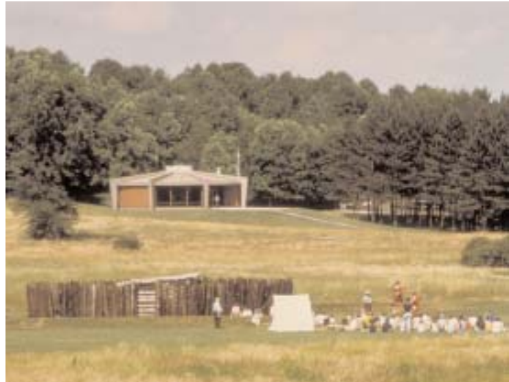
A new visitor center is under construction in a partnership with the Pennsylvania States Heritage Parks Program. It will replace the current outdated center and feature an exemplary interpretive facility for park visitors.
