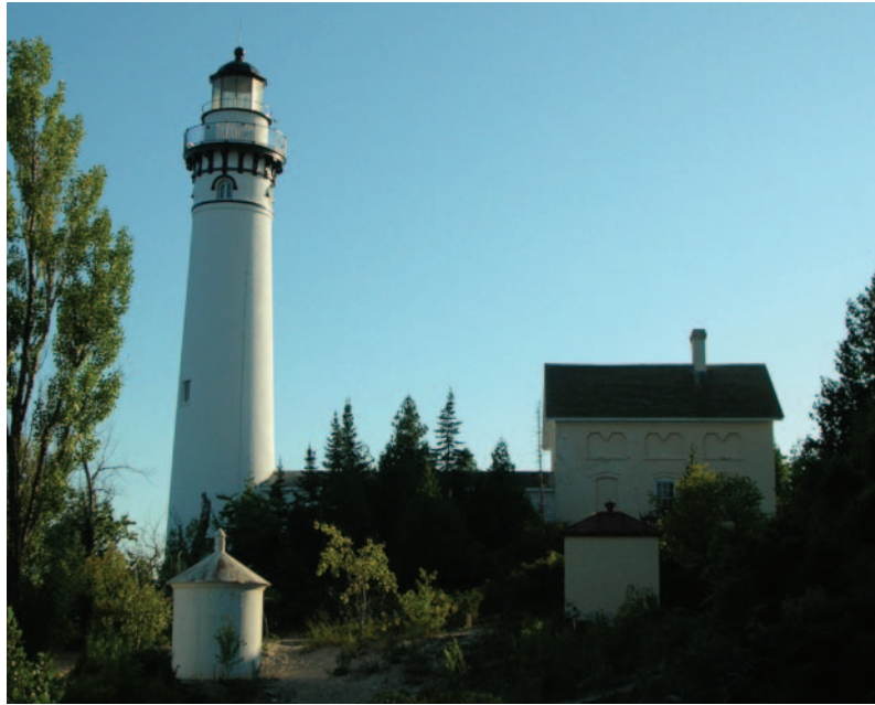
Visitors can climb to the top of the historic South Manitou Island Lighthouse.
