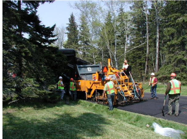
Road rehabilitation in Acadia National Park. © NPS
