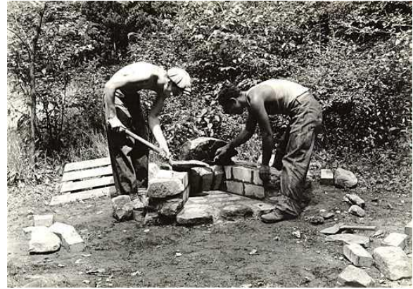
Members of the Civilian Conservation Corps construct a fireplace in a picnic area in Morristown National Historical Park in New Jersey. Photo circa 1935; courtesy of National Park Service Historic Photograph Collection.
