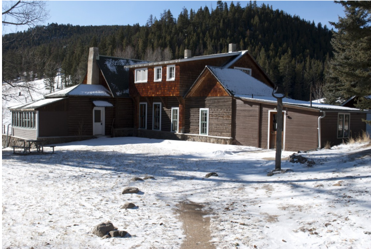
Continental Divide Research and Learning Center, Rocky Mountain National Park. The main building at McGraw Ranch was completely rehabilitated with funds, staff, and volunteers from the National Trust for Historic Preservation and NPS to provide kitchen, meeting, sitting, and office space for park staff and visiting researchers. Credit: Dan Saxton.
