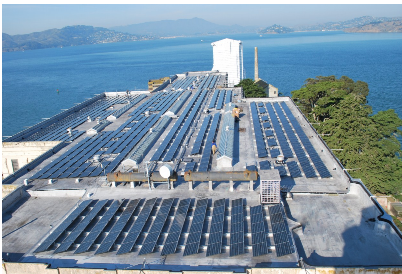
Golden Gate National Recreation Area recently installed a solar array on the roof of the Main Cell Block at Alcatraz Island, a National Historic Landmark. This modification helps to eliminate the use of fossil fuel generators on the island. By installing the solar panels in a low-profile configuration hidden from ground-level view by the roof parapet, this project took advantage of the building’s historic features instead of compromising them. Credit: Don Mannel/ National Park Service.
