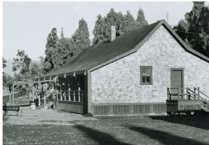
Volcano House after rehabilitation. Credit (top and bottom): National Park Service.
