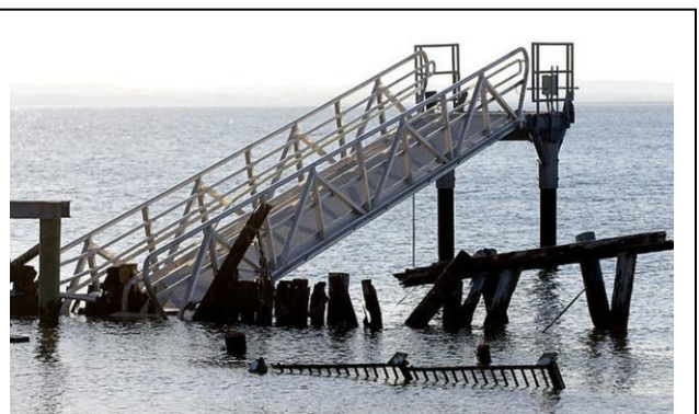
Storm damage to ferry terminal at Sandy Hook
