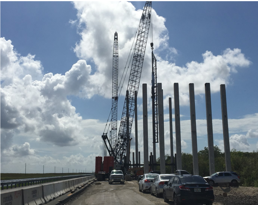
Tamiami Trail 2.6 mile bridge construction, June 2017. Photo: Cara Capp, NPCA
