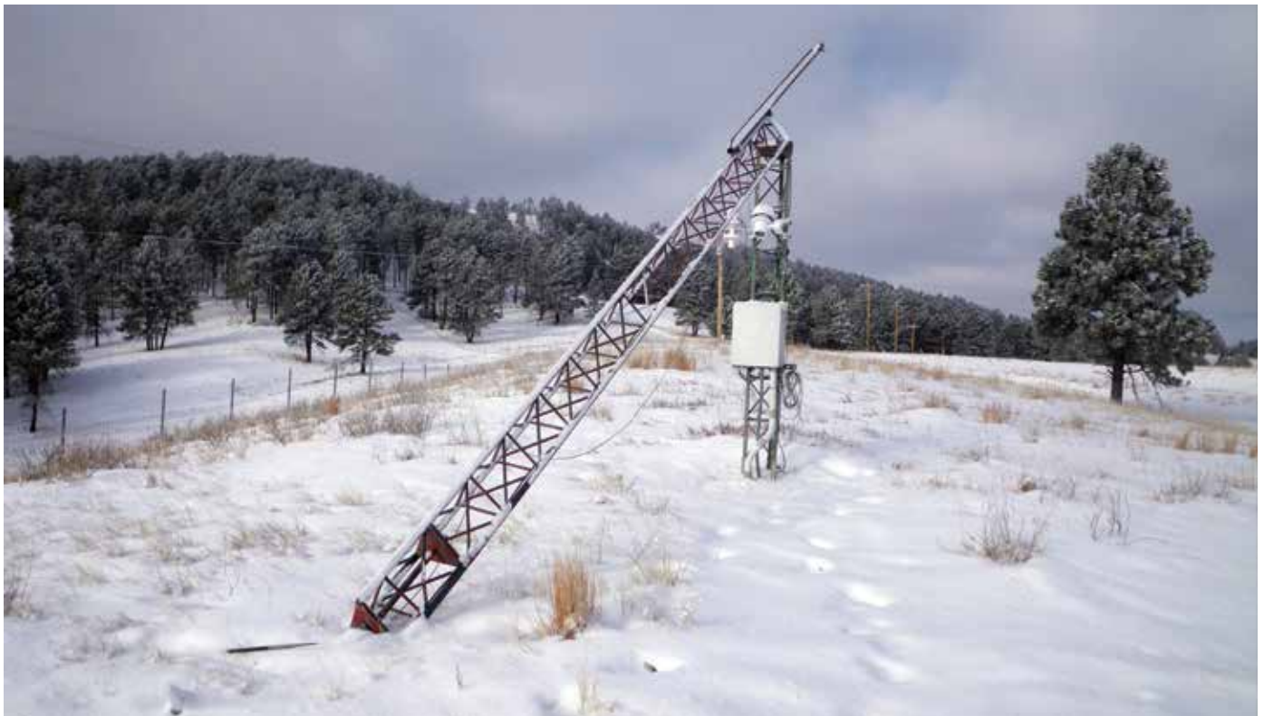
Below: Air monitoring tower at Wind Cave National Park broken during a strong blizzard in December 2017 ©National Park Service
